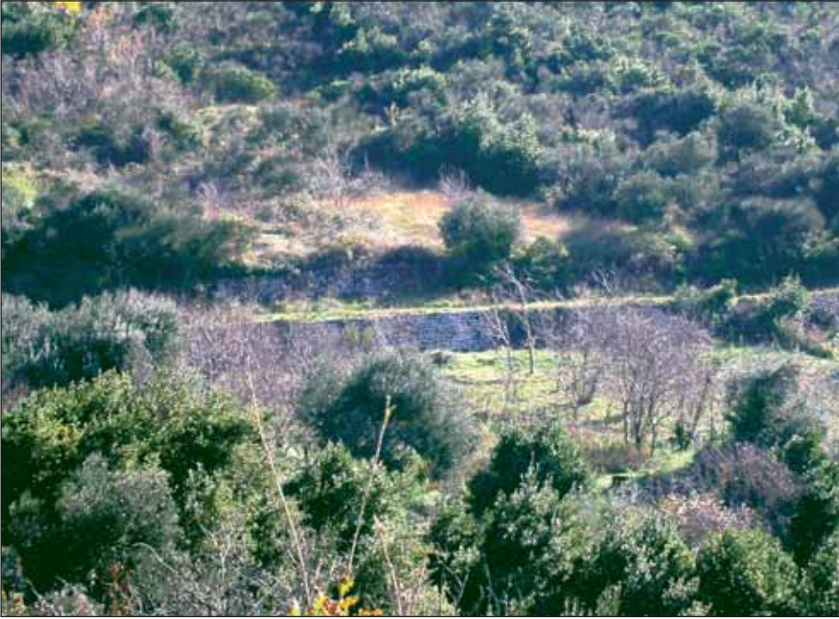
Figure 5: Initial part of the aqueduct route on flyschy terrain
