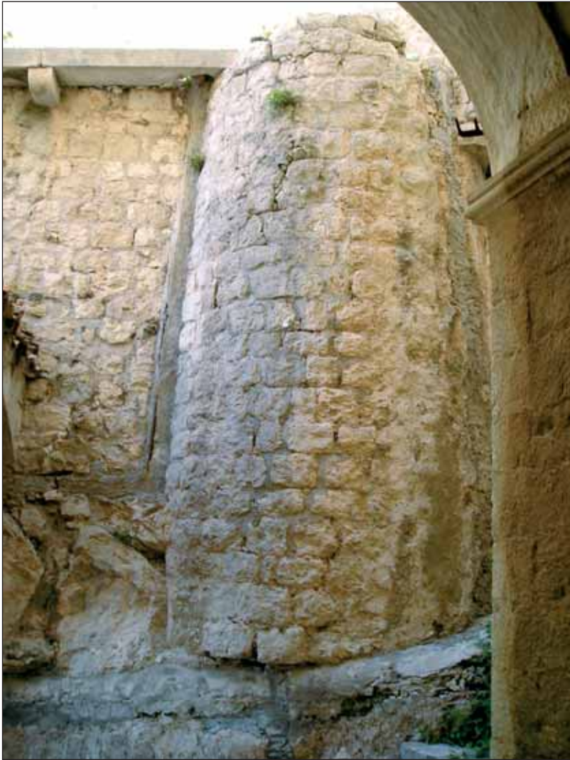
Figure 18: Settling basin within the Franciscan complex
