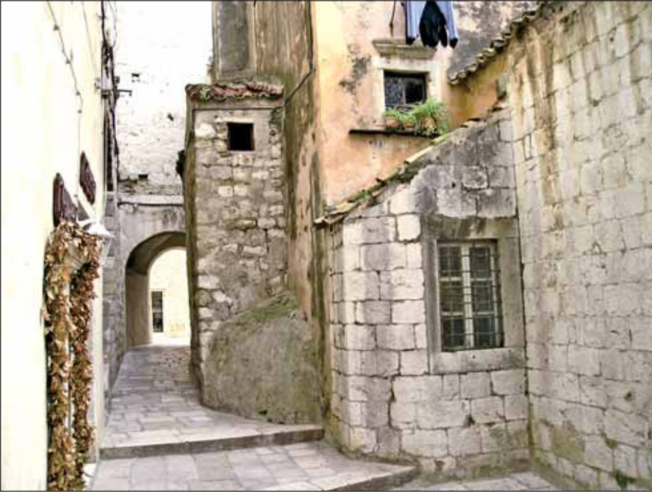
Figure 20: The site of the reservoir ('Depozit'); salt warehouse adjoining the Church of St Nicholas
