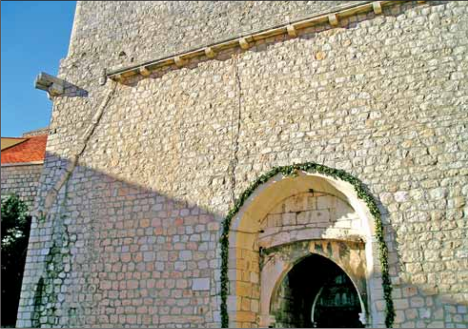
Figure 19: Remains of the canal on the inner side of the city walls that carried water to the Great Fountain
