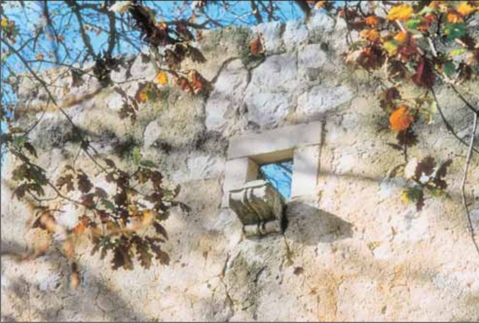
Figure 3. Stone console of the launch opening
