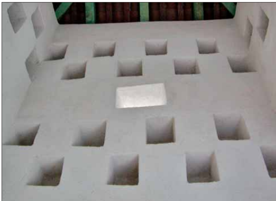
Figure 5. Pigeon holes after the reconstruction
