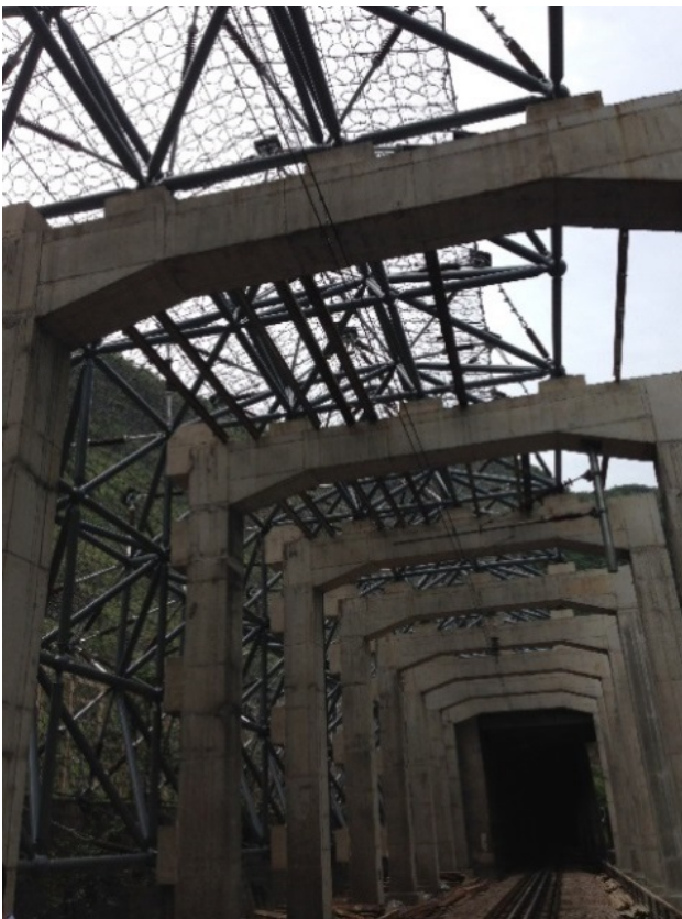
Figure 2. Photo of the finalized structure
