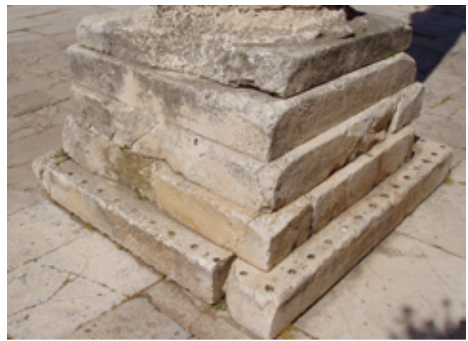
Slika 6. Stepenasta stopa pod bazom kolone na rimskome forumu – raspored utora na donjoj stubi, pogled s istoka Figure 6. Stepped footing under column base on Roman Forum – distribution of grooves on lower step, eastern view
