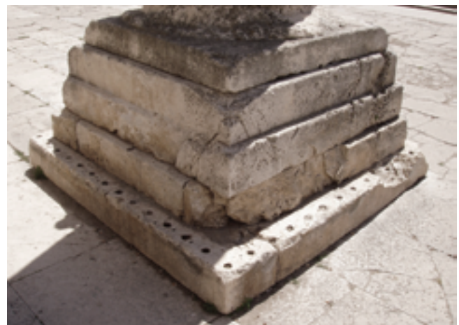
Slika 7. Stepenasta stopa pod bazom kolone na rimskome forumu – raspored utora na donjoj stubi, pogled sa sjevera Figure 7. Stepped footing under column base on Roman Forum – distribution of grooves on lower step, northern view
