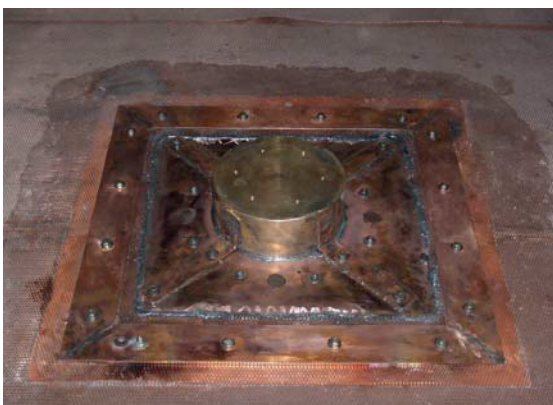
Figure 3. Earth plate electrode
