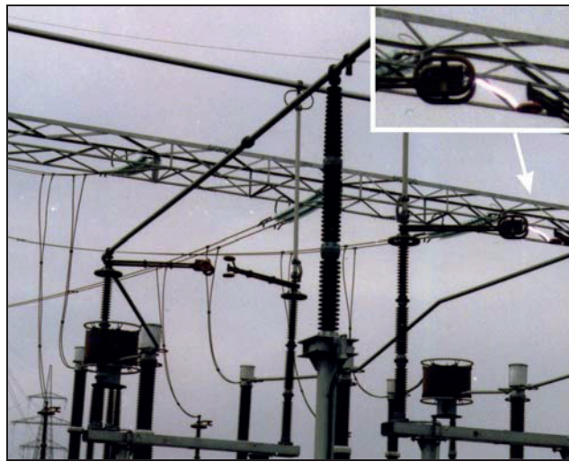
Fig. 1 Arc between contacts of disconnector in AIS 400 kV substation Tumbri, near Zagreb
