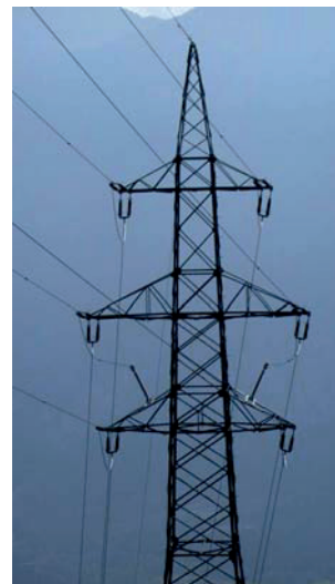
Figure 3: Tower with 2 Line Surge Arresters (Present Situation)
