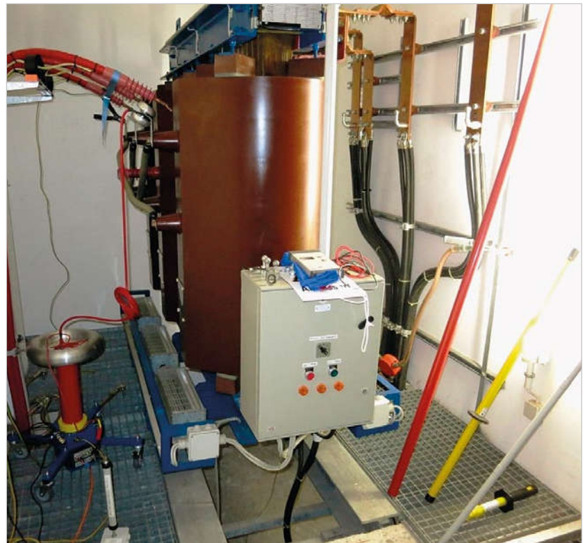
Figure 9. PD measurement setup on a 20 kV / 2 MVA cast-resin transformer
