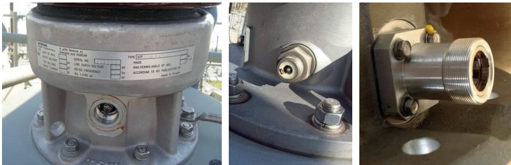
Figure 9 – Different designs of measuring taps (from left to right: Končar OTF type, ABB Micafil type, Passoni-Villa type)
