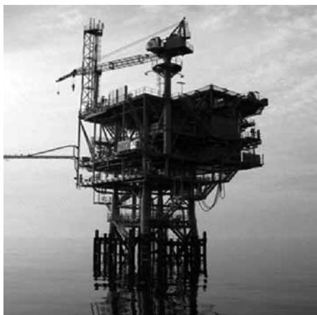
Figure 8 Gas platform Marica
