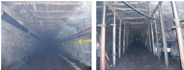
Figure 9 Control effects of the surrounding rocks of the 8105 working face
