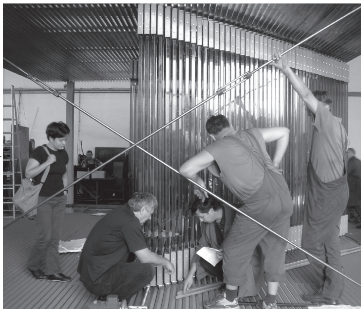
ŠELA WORKSHOP, FRAMEWORKS AT CONSTRUCTION
