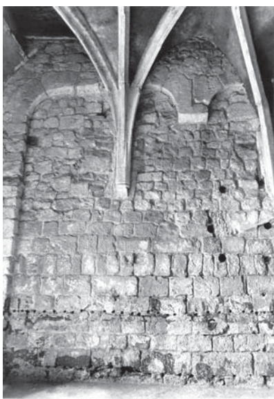
35. Unutrašnjost prizemlja zvonika, pogled na zapadni zid i vratnu nišu nakon odzidavanja / Bell tower ground floor interior, view of the western wall and the door niche after brick de-layering
