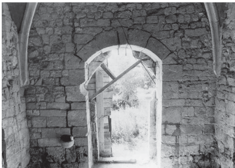
35. Unutrašnjost prizemlja zvonika, pogled na zapadni zid i vratnu nišu nakon odzidavanja / Bell tower ground floor interior, view of the western wall and the door niche after brick de-layering
