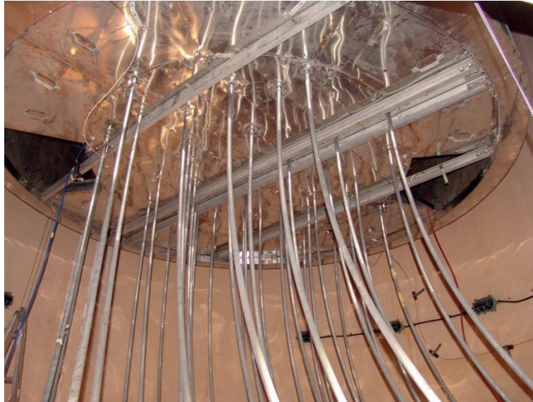
Figure 7: NPP Krško RPV insulation details (1) - inspection openings
