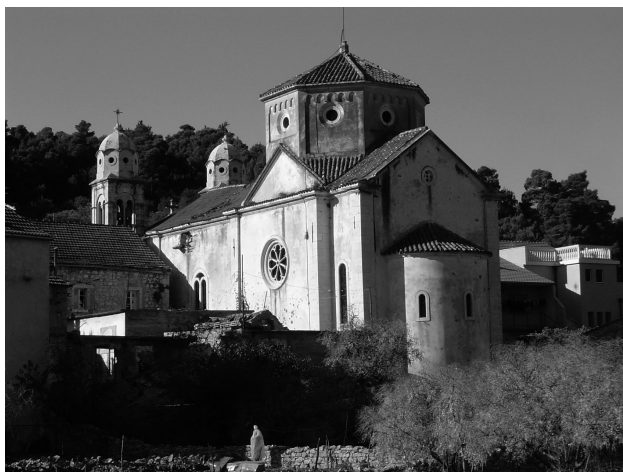
1. Crkva sv. Spiridona, pogled s jugoistoka / Church of St Spyridon, view from southeast /
