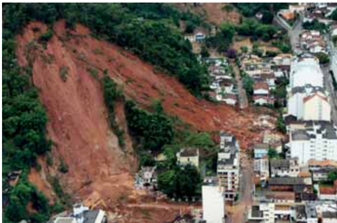
Figure 1. Landslides effects on electric power facilities [1]
