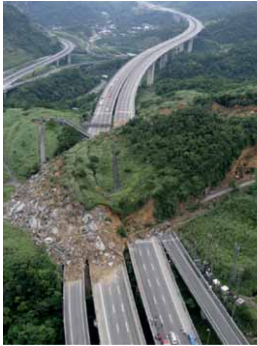
Figure 3. The impact of landslides onto the highway [1]
