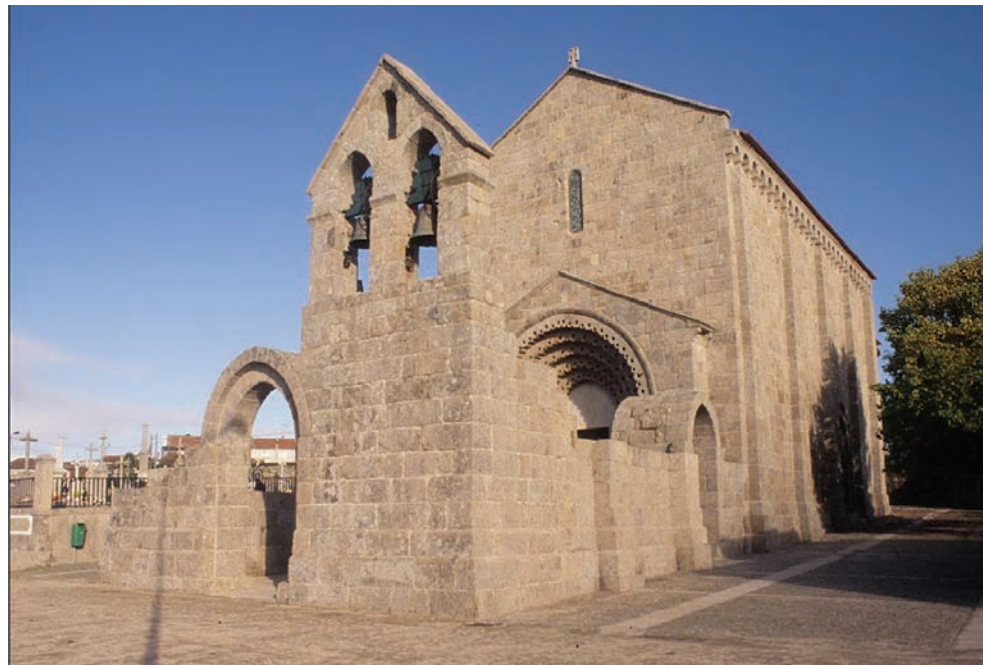
Fig. 7 - São Pedro of Ferreira, Paços de Ferreira, Portugal, church and the misinterpreted of the former galilee, unroofed
