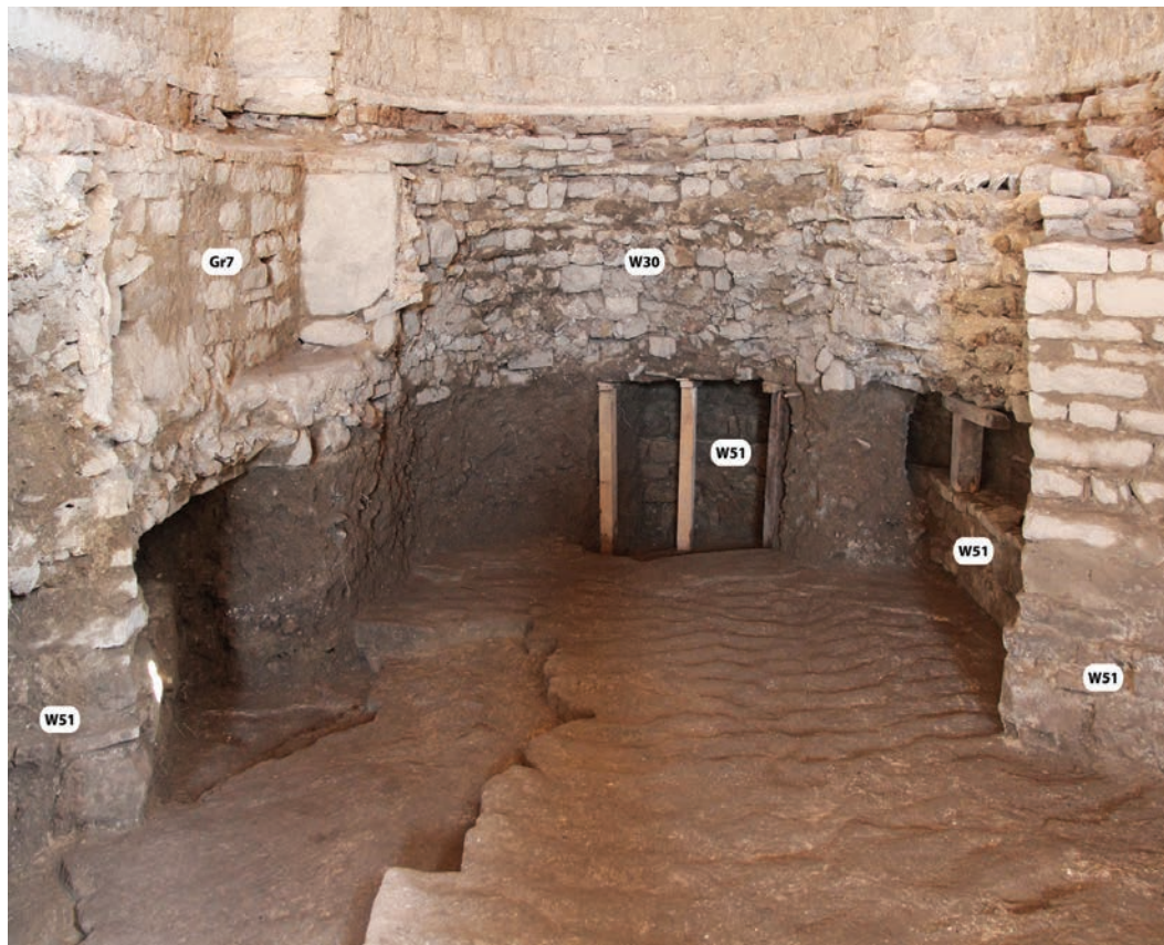
Fig. 13. Trench T10 after excavation; view SE (A. Milošević).
