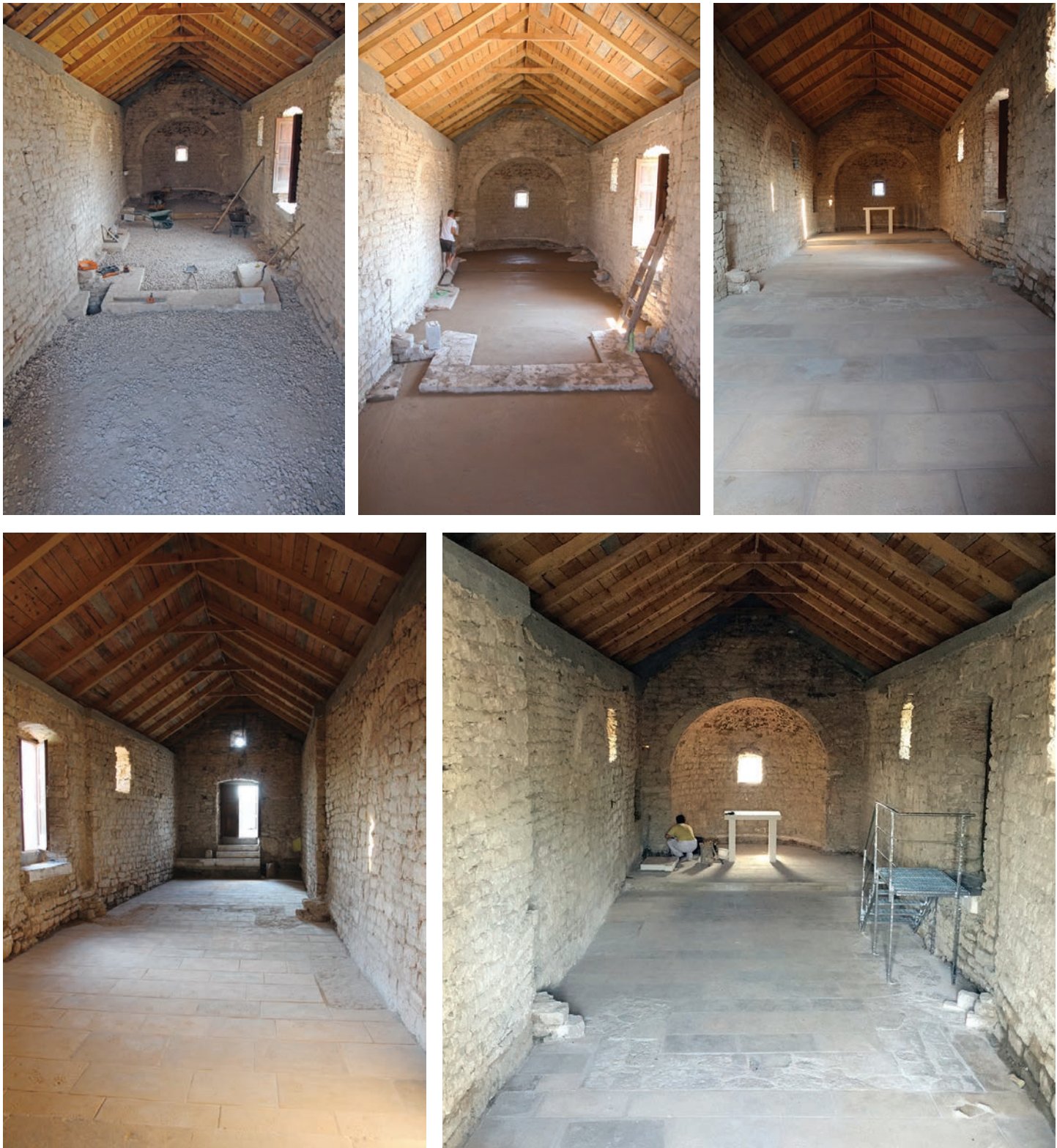
Fig. 38. Different stages of the reconstruction of the subfloor and floor levels in the church of Sts Joachim and Ann (A. Milošević).
