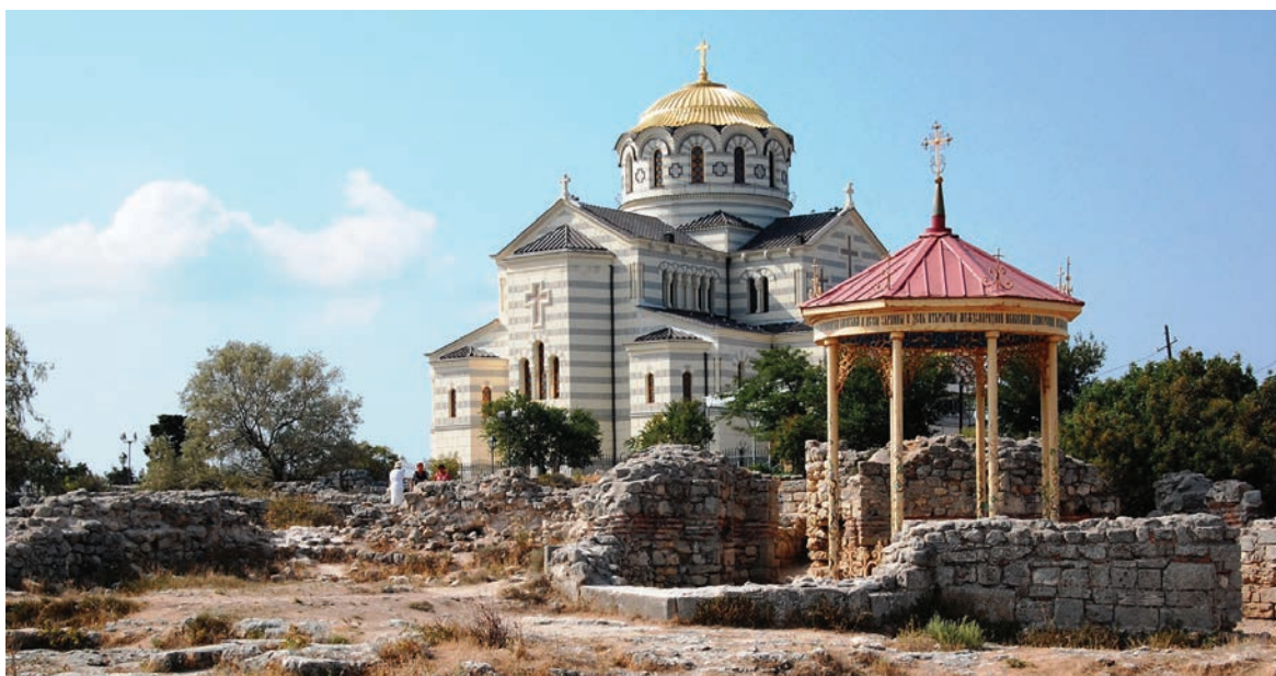
Fig. 5. Complex of Uvarov's basilica. Baptistry, view to the South (photo L. Khrushkova)
