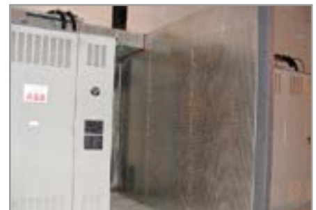
Figure 8. Critical equipment separation wall
