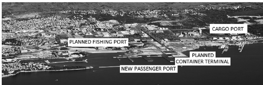
Figure 5 - The envisaged construction area for the fishing port and container terminal in the Port of Gaženica [authors]
