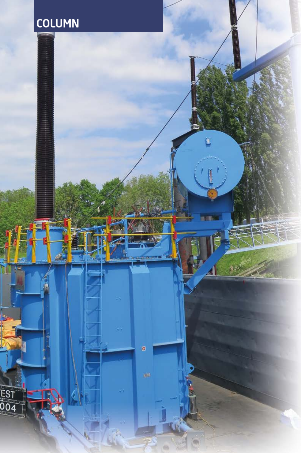
Figure 1. Preparation of a 765 kV transformer prior to short-circuit test in a barge at KEMA Laboratories at DNV GL
