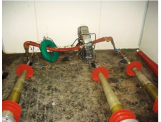
Figure 3. Low temperature test with current injection
