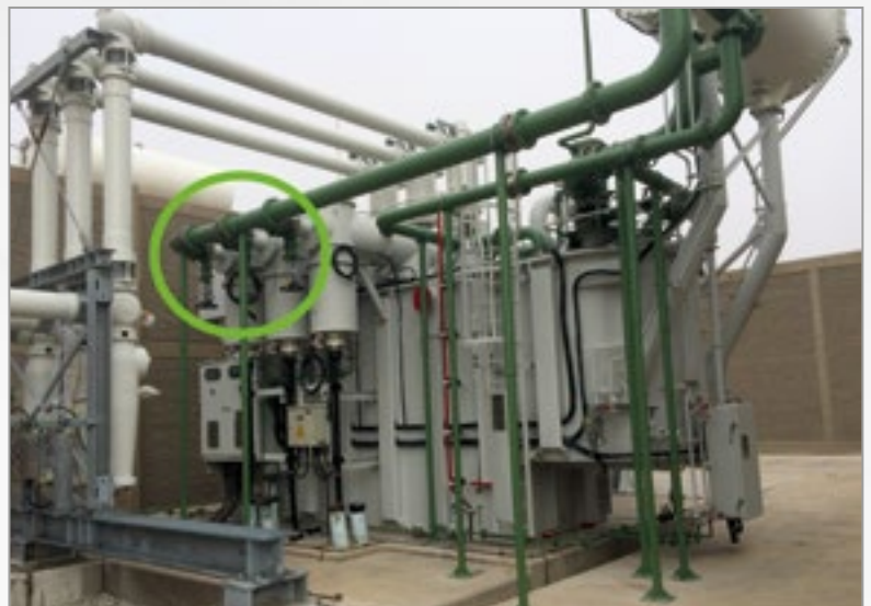
Figure 2. Installation of a transformer fast depressurization system, including bushing turret protection
