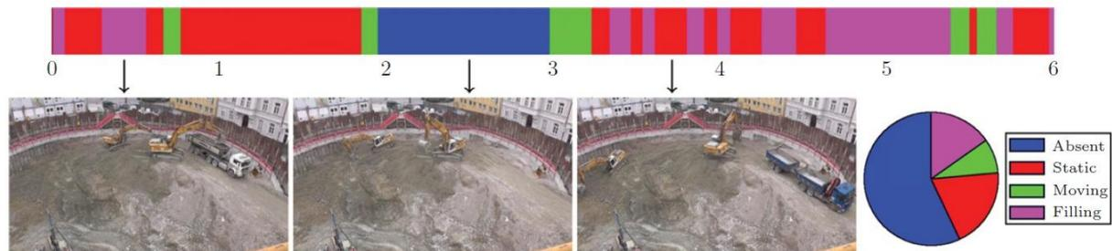
Figure 3. An example of dump truck activities in a video segment of 6 minutes duration (taken over: Bügler *et al.*, 2017)
