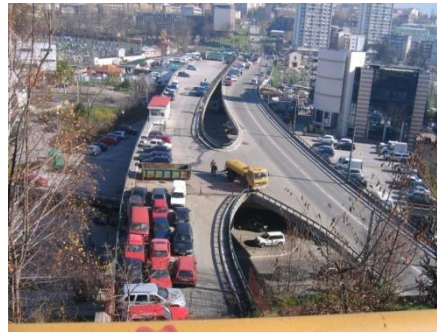
Figure 3 – Present state of the Koševo viaduct
