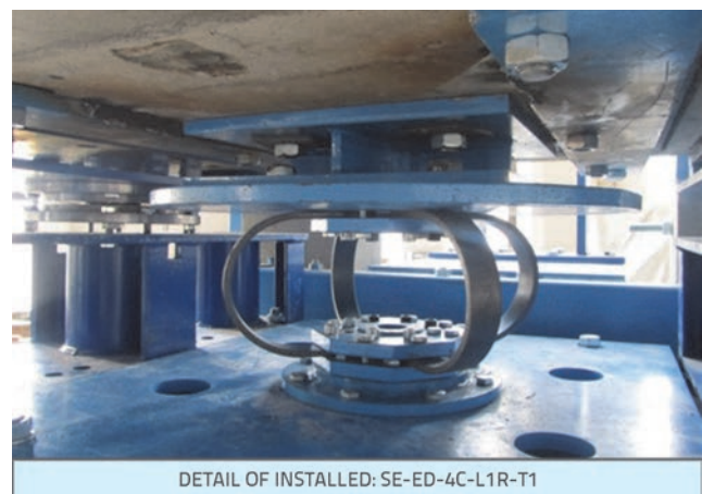
Figure 20. Constructed and installed set of two DSRSB devices and one SF-ED-4C-L1R-T1 device at right end support of the tested bridge prototype model
