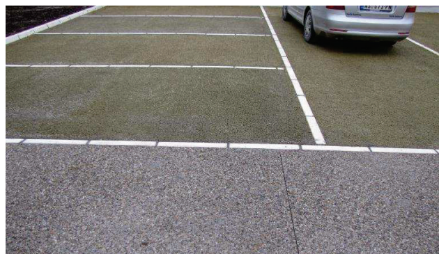
Figure 17 Application of pervious concrete in Serbia
