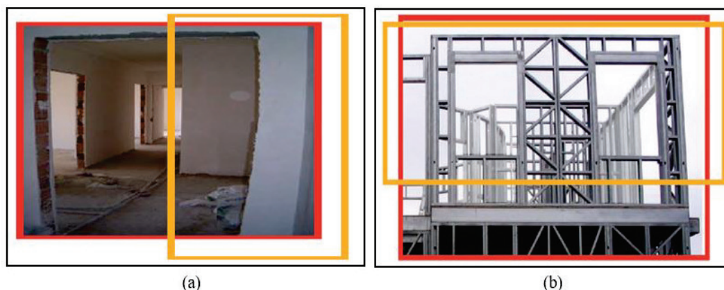
Figure 4 (a) Door frames' accuracy error for reinforced concrete structure, (b) Door frames' exact accuracy for lightweight steel structure
