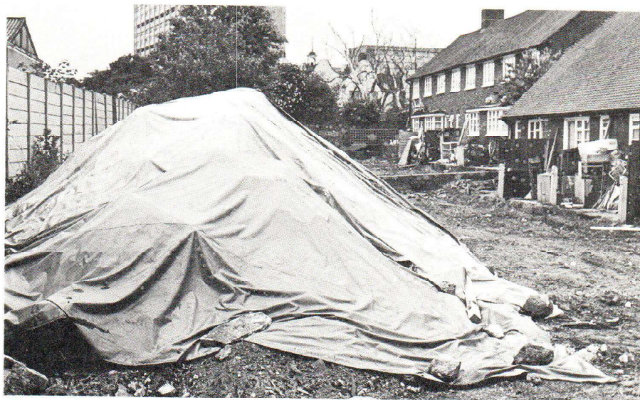
FIG. 1 — Tarpaulin covered mounds of asbestos-contaminated soil in the gardens of houses at Barking.
