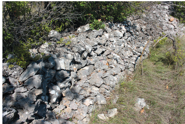
Fig. 7. The layers of the enclosure (photo: N. Cesarik).
