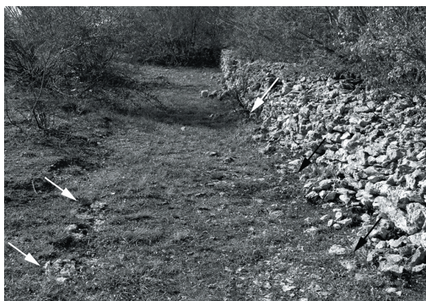
Fig. 11. The kerbs of the Roman road towards the river Cetina (photo: N. Cesarik).
