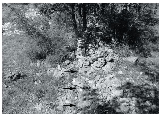
Fig. 8. The remains of a foundation of the wall (photo: N. Cesarik).
