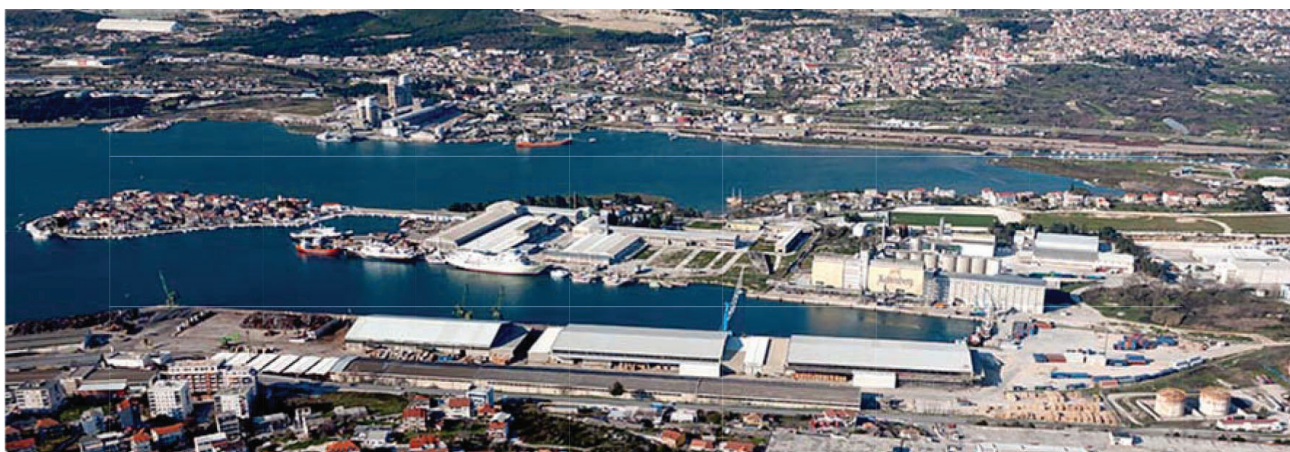
Figure 1 North Port of Split – modified [20]
