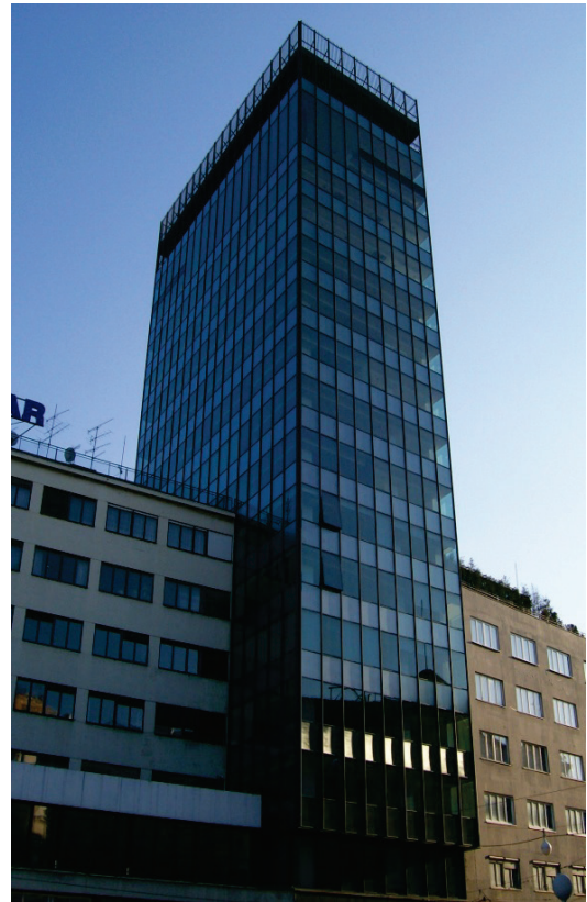
Figure 12 Skyscraper in the Ilica street - photo
