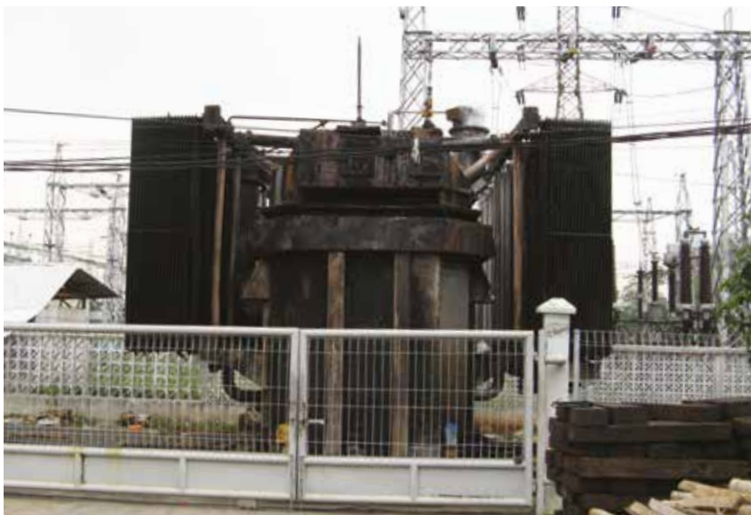
Figure 2. Failed transformer
