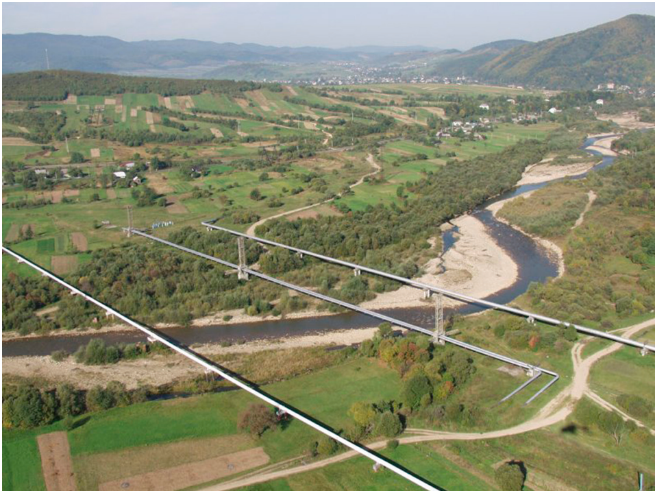
Fig. 1. An above-ground gas pipeline with diameter 1420 mm. The Carpathians, Ukraine (UKRTRANSGAZ 2015).
