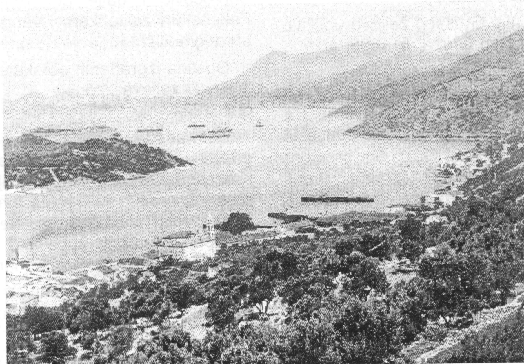
Slika 7. Slika krajem 19. stoljeća – izgrađen je gat “Petka”, a na ostalom prostoru zaljeva uočljiva je prirodna obala Figure 7. Photo from late 19 th century – the jetty “Petka” was built. Natural coast can be noted in the remaining space of the bay.
