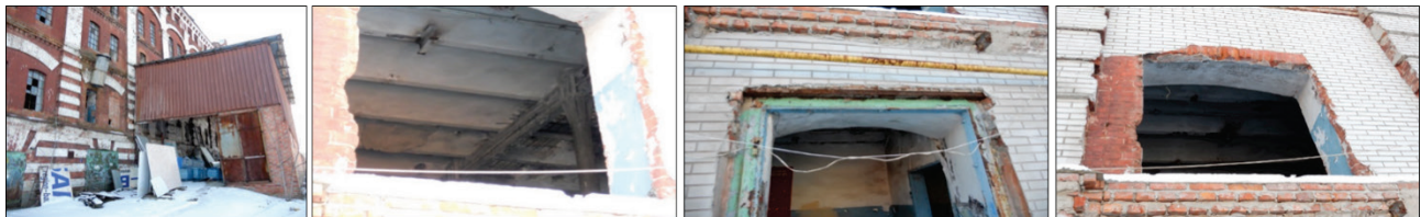
Figure 2 Physical conditions of the building
