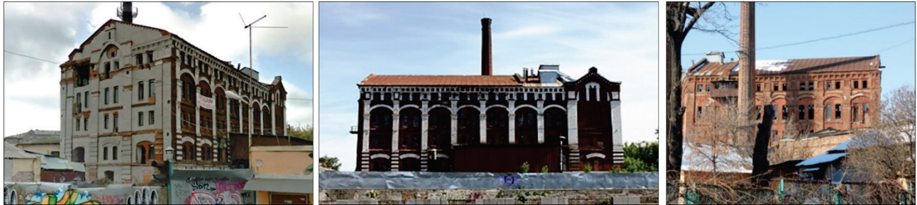
Figure 1 The old mill building
