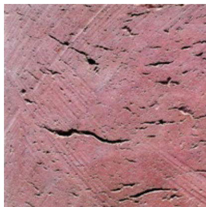
Figure 8 Internal cracks in a cube cut in a section perpendicular to casting layers
