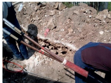
Image 13 Making of cable joint
