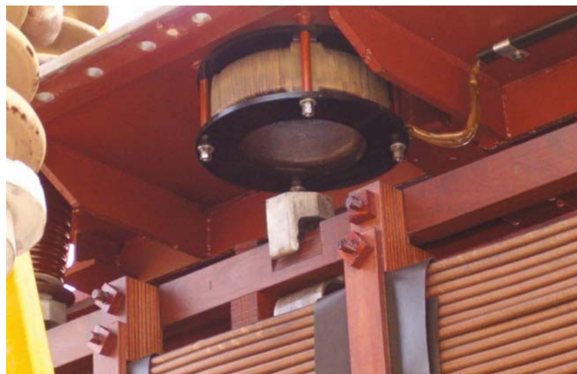
Figure 11. A case of internal failure occurring at gas concentrations of 800 ppm hydrogen and 55 ppm methane
