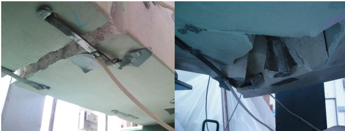
Figure 10. Cramps and dowels pulling out from their seats
