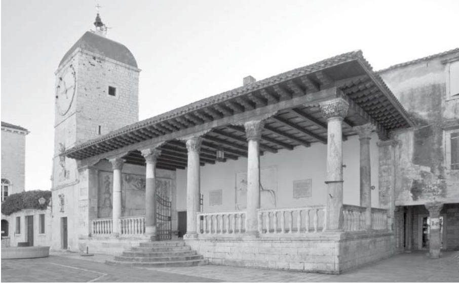
Figure 7. Loggia (photo by Joško Ćurković)
