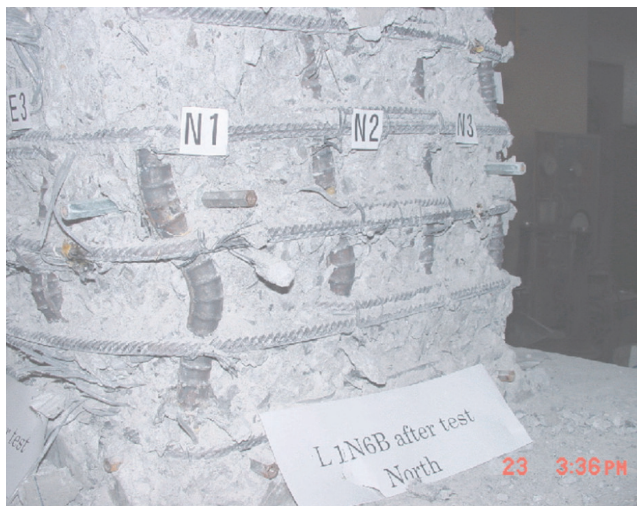
Figure 13. Expansion of shear reinforcement and crashing of corners concrete [17, 18]
