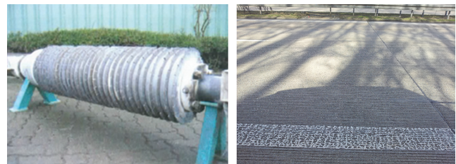
Figure 19. Grinding grooves on roadway surface
