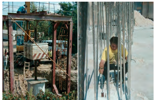
Fig. 1. Dynamic testing of the pile capacity and integrity of pile columns
