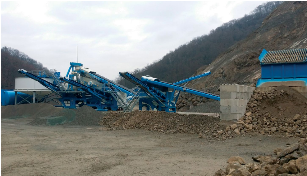
Fig. 3 – Semi-mobile processing plant M2500 E5X
