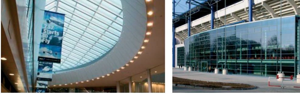
Fig. 22 – Examples (14), a) The roof of Terminal 1, Narita International Airport, Tokyo, Japan, b) MSV Arena Soccer Stadium with Pilkington glass facade, Duisburg, Germany
