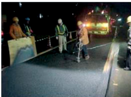
Fig. 12 – The use of \text{TiO}_2 photocatalytic material on a pavement structure for the purpose of reducing pollution in Japan, a) application of coating b) pavement structure with the lighter part where coating has been applied (22)
