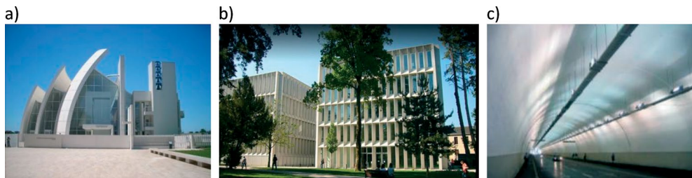
Fig. 10 – a) Church Dives in Misericordia in Rome, Italy (14), b) Music and Art City Hall , Chambéry, France, (15), c) Umberto tunnel I , Rome, Italy (15)
