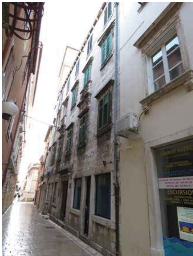
3. Kuća Dragičević–Pappafava, pročelje Dragičević–Pappafava House, front façade
