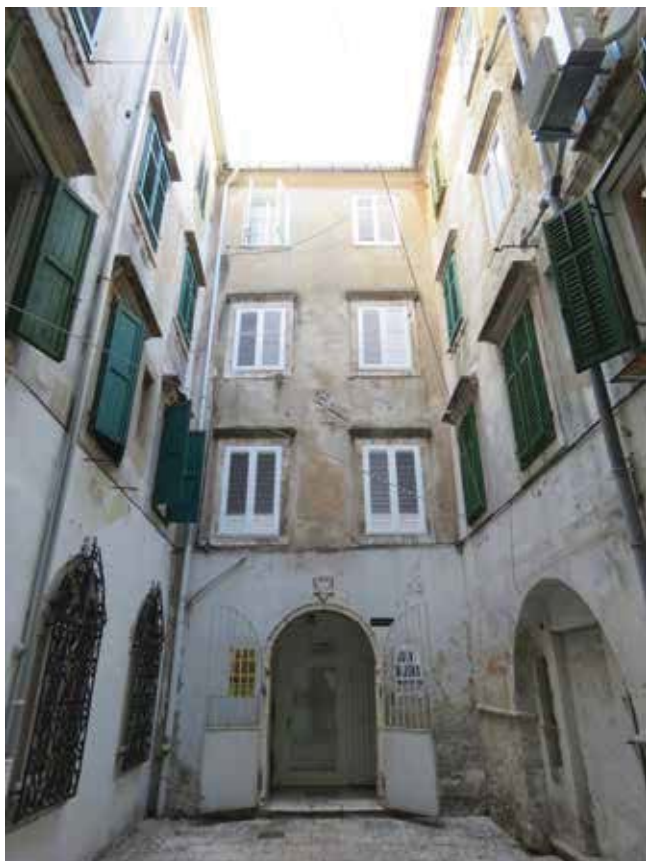
8. Središnji dio kuće Dragičević–Pappafava s portalom i grbom, pogled iz unutarnjeg dvorišta Central part of the Dragičević–Pappafava House with a portal and a coat-of-arms, view from the inner courtyard
