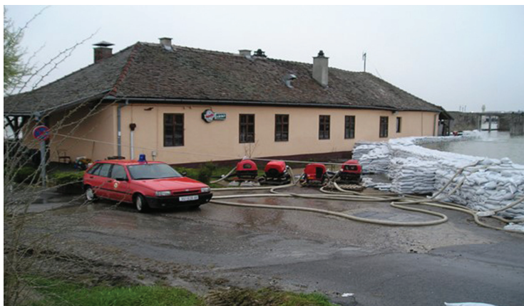
Slika 3. Zečji nasip i ispušavanje vode Dunav, Vukovar 2006. godina Figure 3. The boulder and pumping water of the Dunav, Vukovar 2006
