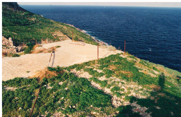
Fig. 9. The water pipe system of the Yugoslav Army (photo: Kirigin 1992)
